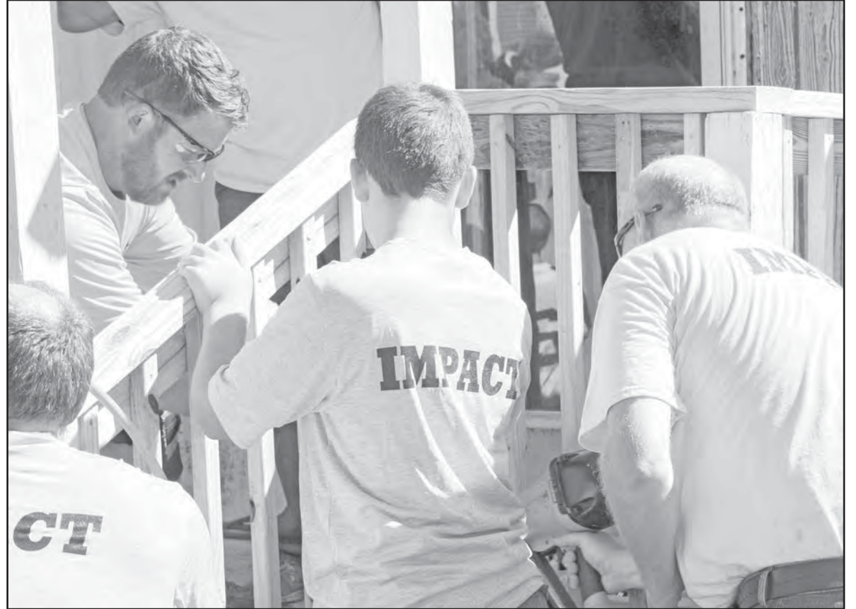
The Impact Project volunteers help people with anything from new wheelchair ramps to new roofs at no cost to the beneficiary. (Photo by Zachary Meseck)
