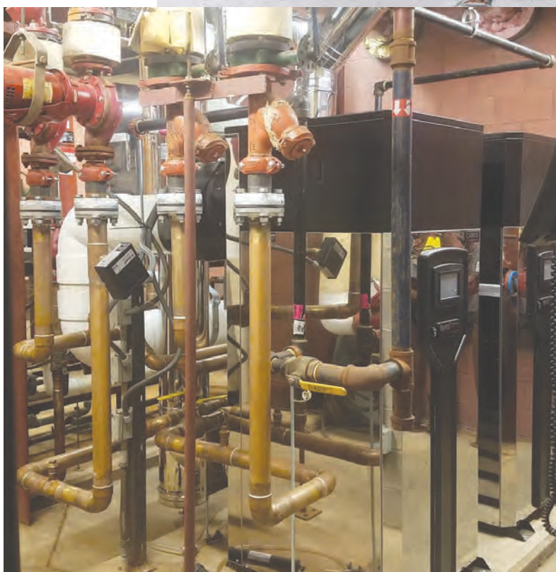
The Norwich Family YMCA installed a new five boiler system with 95 to 96 percent energy efficient water boilers, and made it so the system could swap between them when one needs maintenance. (Norwich Family YMCA photo)
