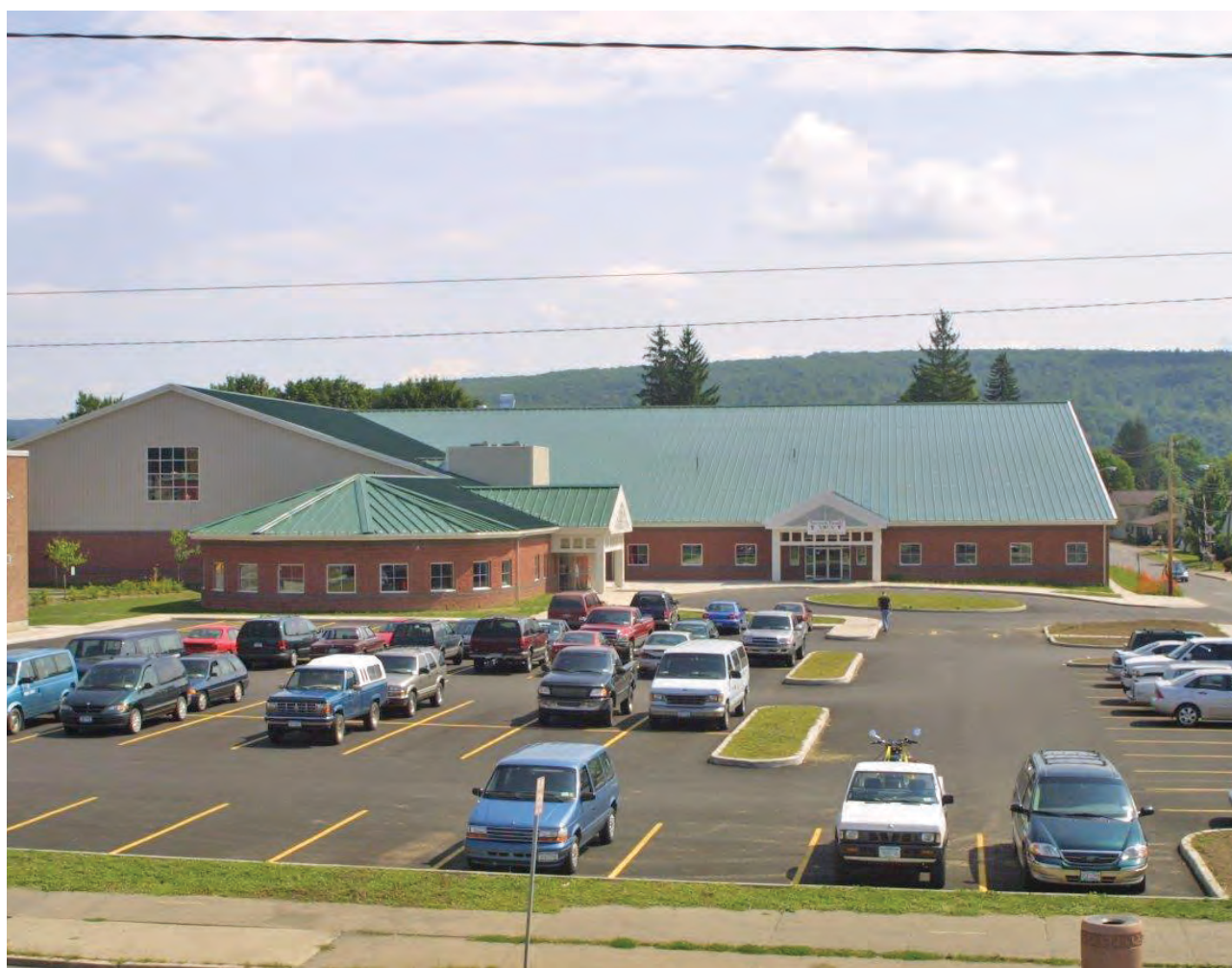
2018 was a year of investment for the Norwich Family YMCA, with replacements to floor tiling, countertops, and upgrades to security. (Frank Speziale photo)
