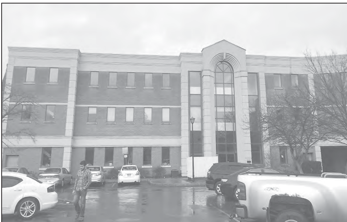
A view of the backside of the building Principle Design & Engineering, PLLC, will renovate into a new hotel.
