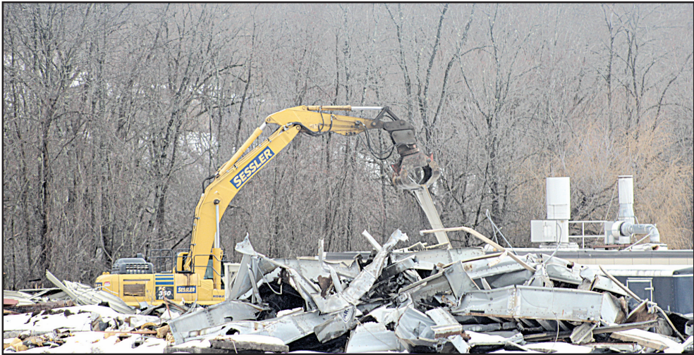
An excavator demolishes one of the industrial buildings once located at Woods Corners in Norwich in this photo from December, 2025. The site is now one of several brownfield areas in Chenango County that may benefit from new study being pursued by the Chenango County Industrial Development Agency. (Photo by Shawn Magrath).
