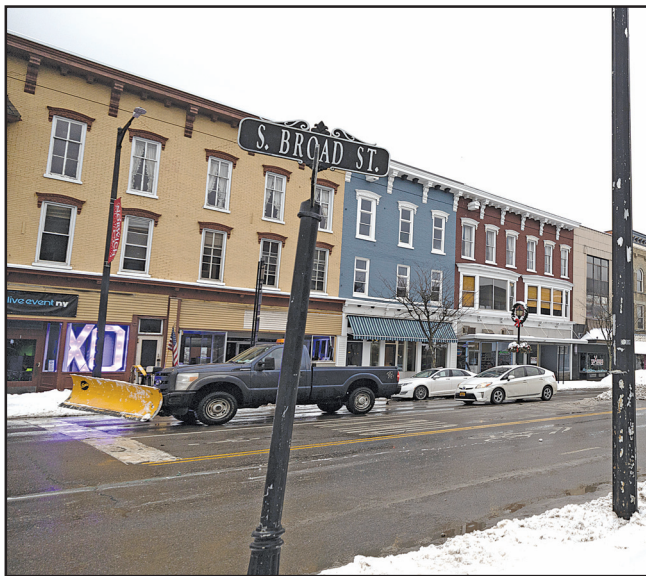
The City of Norwich is preparing to begin work on the placemaking initiative, which will use smaller improvement projects to tie together the larger projects included in the DRI. (Photo by Sarah Genter)
