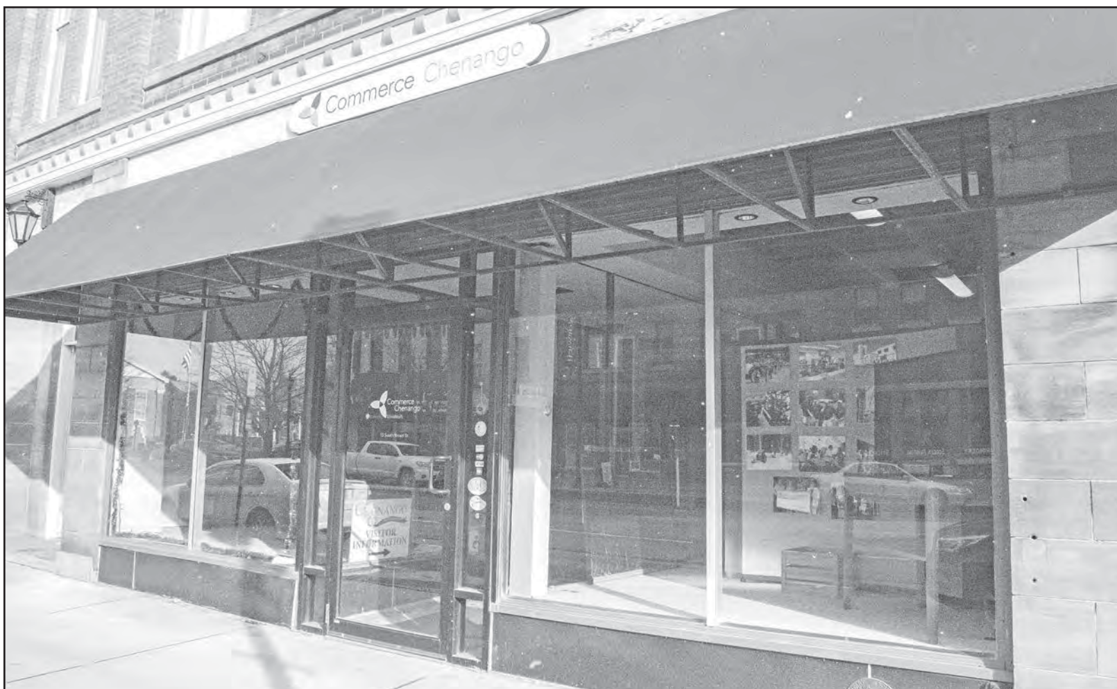
Commerce Chenango's Headquarters is located on 15 South Broad Street in the City of Norwich. (Photo by Zachary Meseck)
