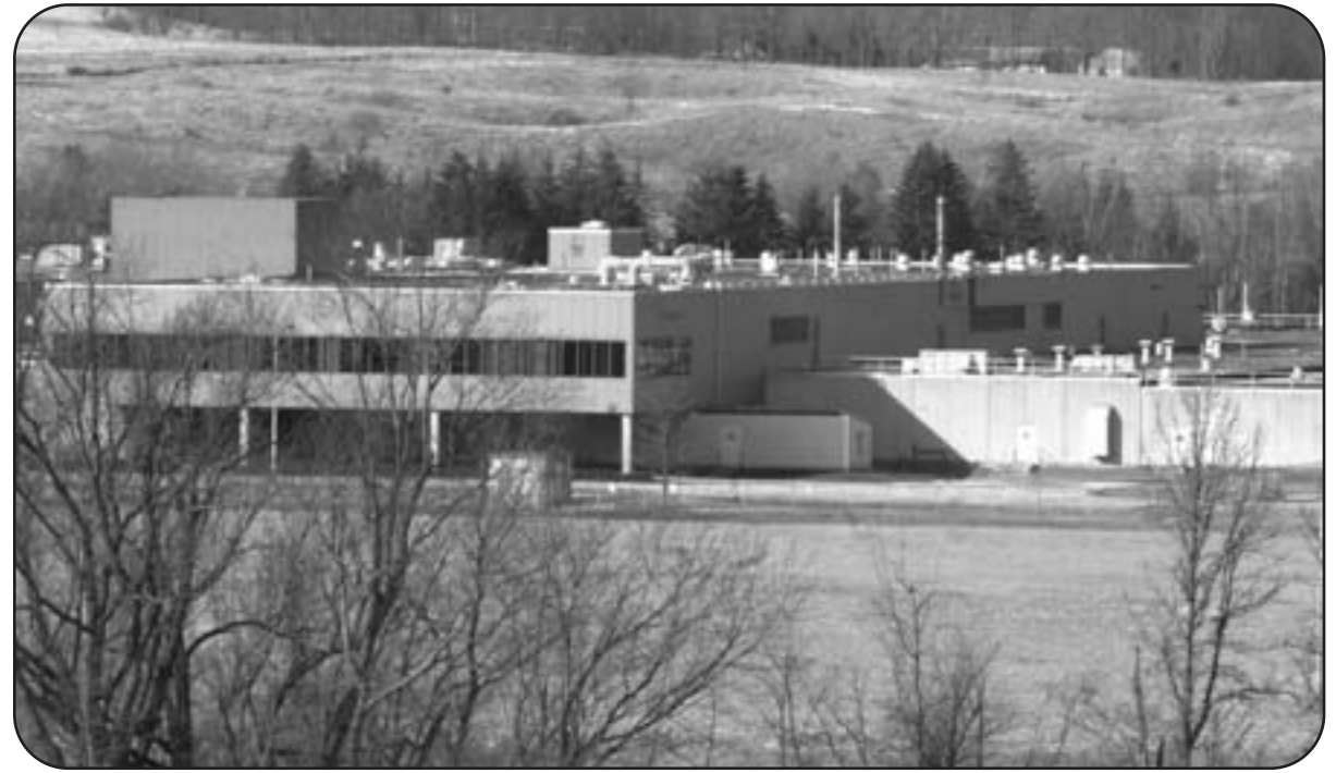
Norwich Pharmaceuticals saw a year of new equipment investments and capability in 2009 and hopes to reap their rewards in 2010. (Photo by Frank Speziale)
